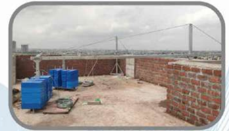
Terrace boom set with counter weight
